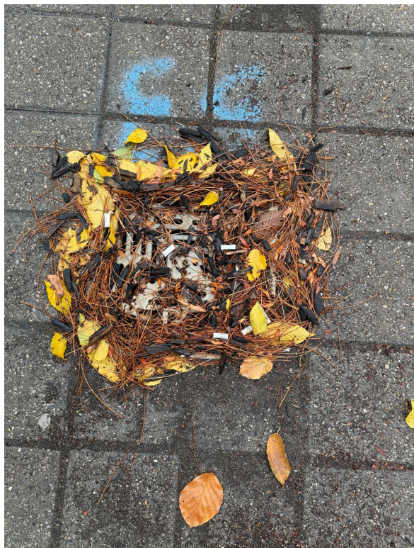
Figure 8. Blocked drain.
