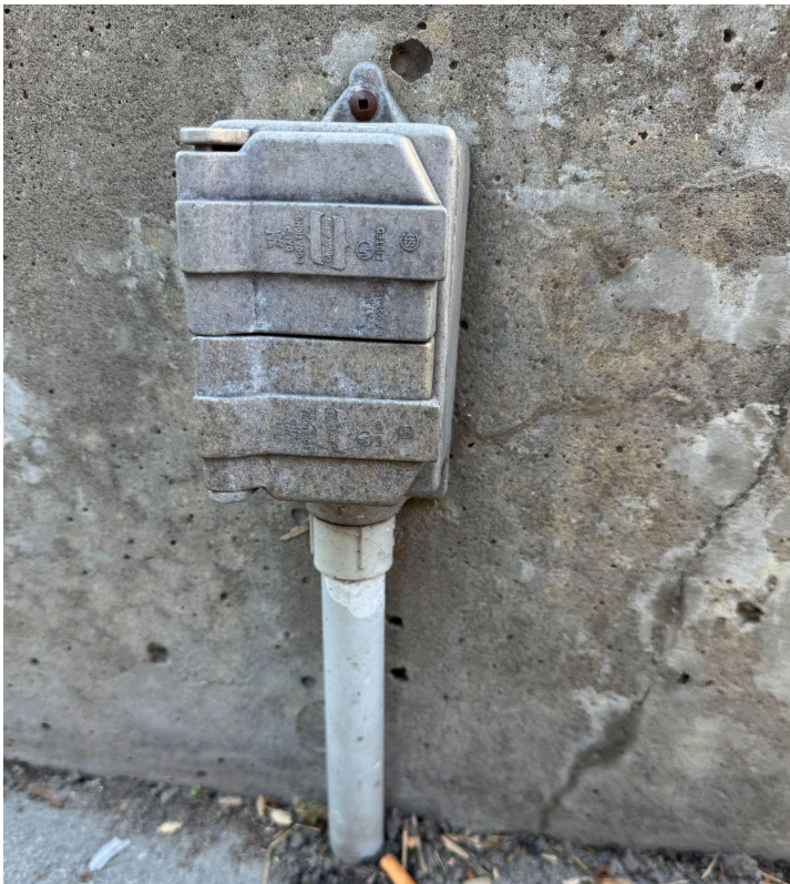
Figure B6. Electrical receptacle (GFCI outlet) with weatherproof cover for outdoor Courtyard.
